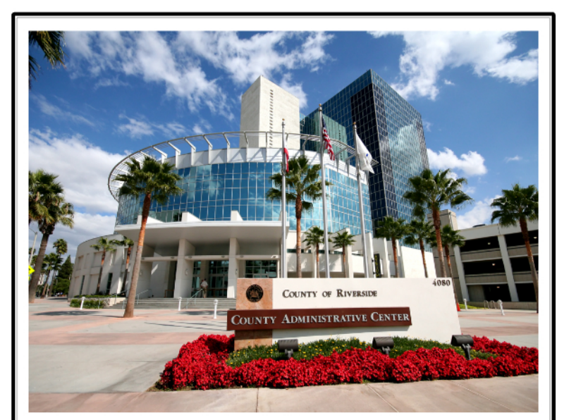
County Administrative Center
